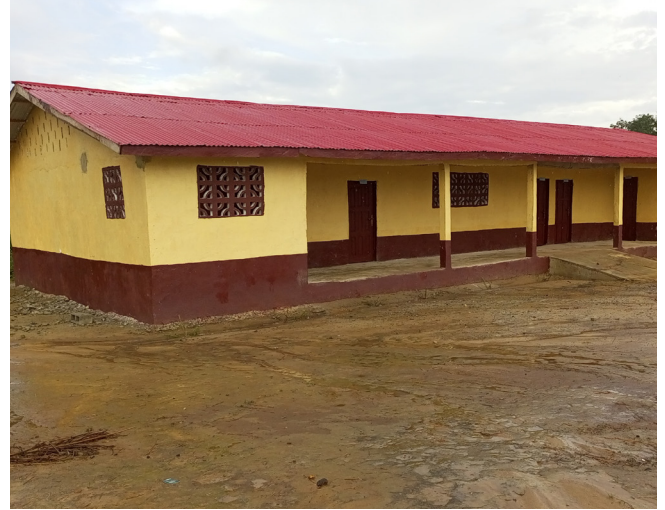
Safe Home: Finished School Building.
